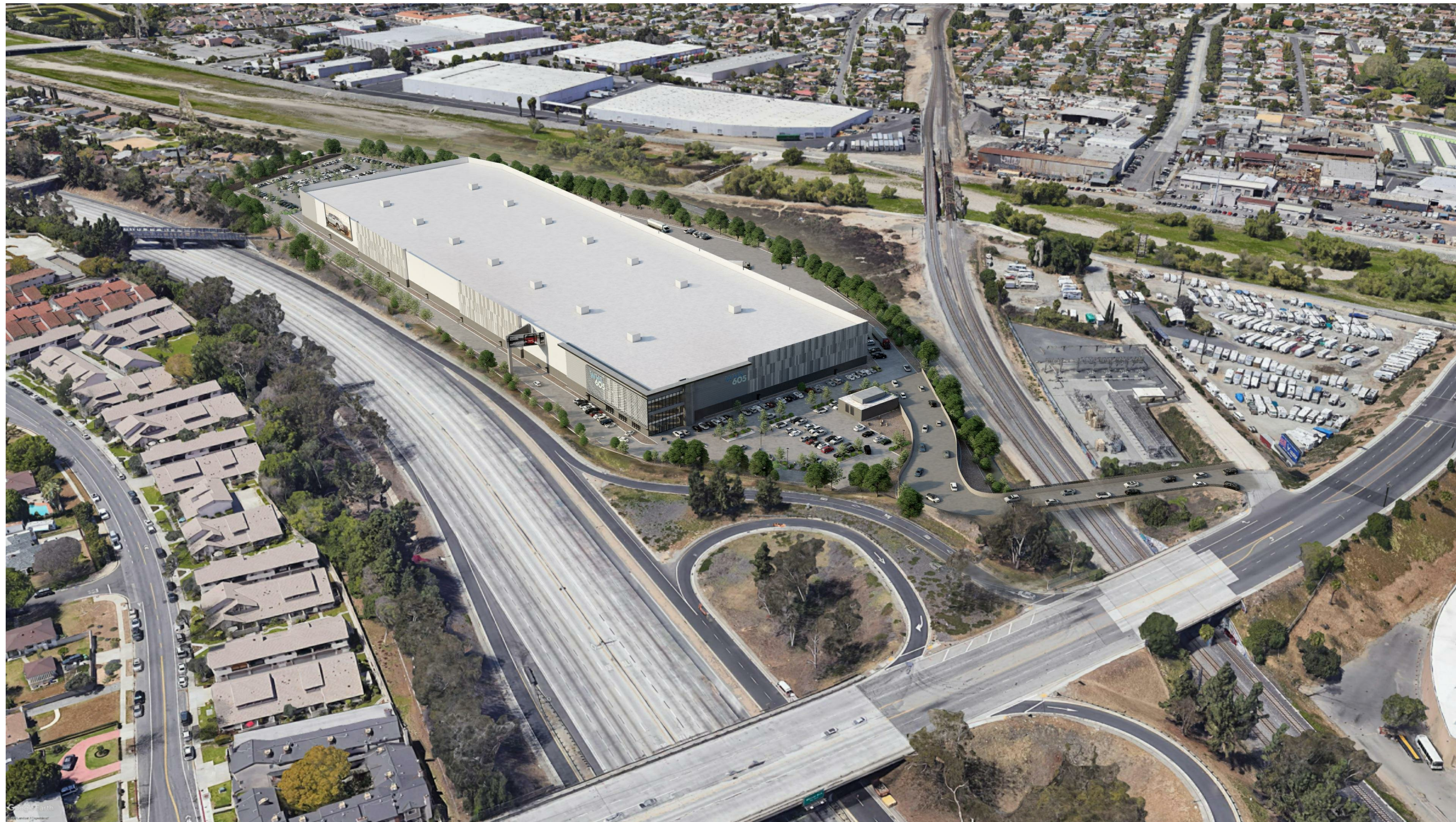
AERIAL VIEW - OVERALL PROJECT
