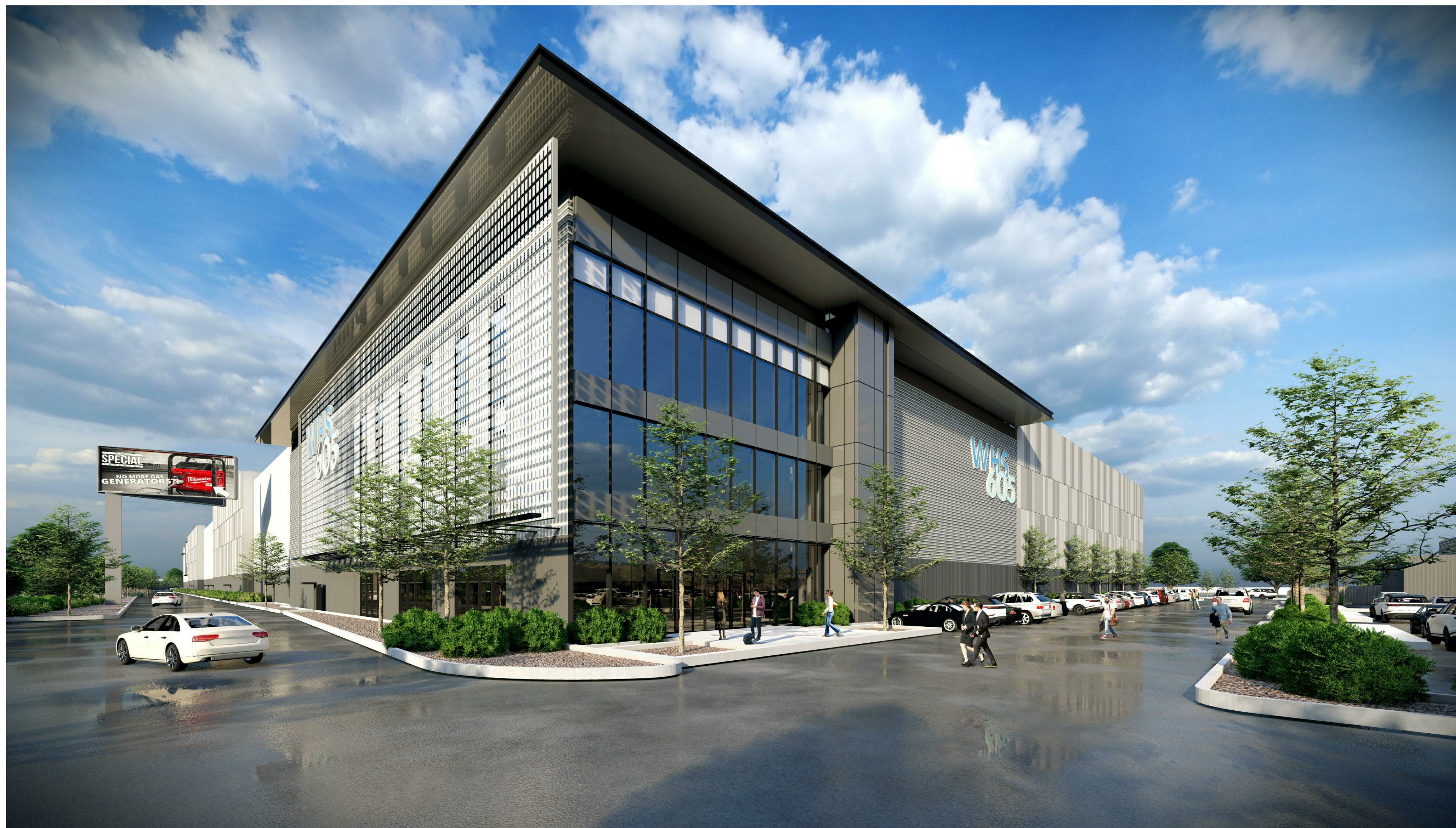
INDUSTRIAL BUILDING - NE CORNER OFFICE ENTRANCE
