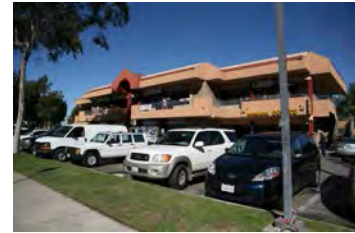
Existing two-story commercial building
