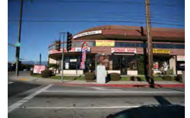
Existing building at the northeast corner of Beverly Boulevard and Rosemead Boulevard
