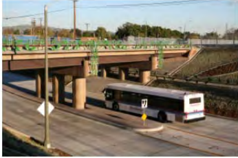
View of the Passons underpass
