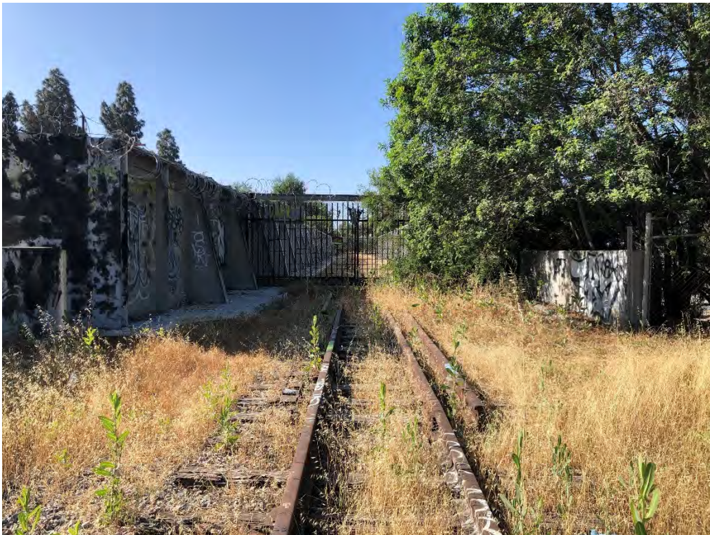
Photograph 10: Standing in the southeastern corner of the project site, facing south towards the former railroad spur that extends across I-605.
