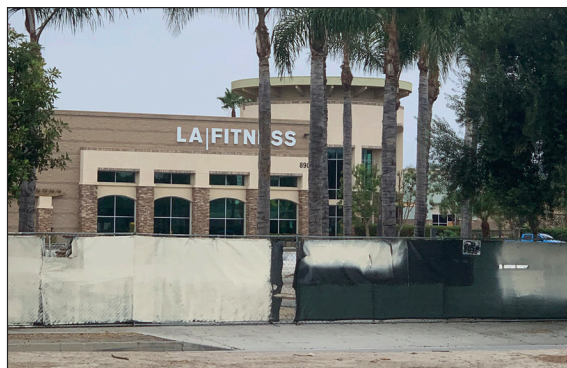
View to site and LA Fitness from the South/Washington Blvd.
