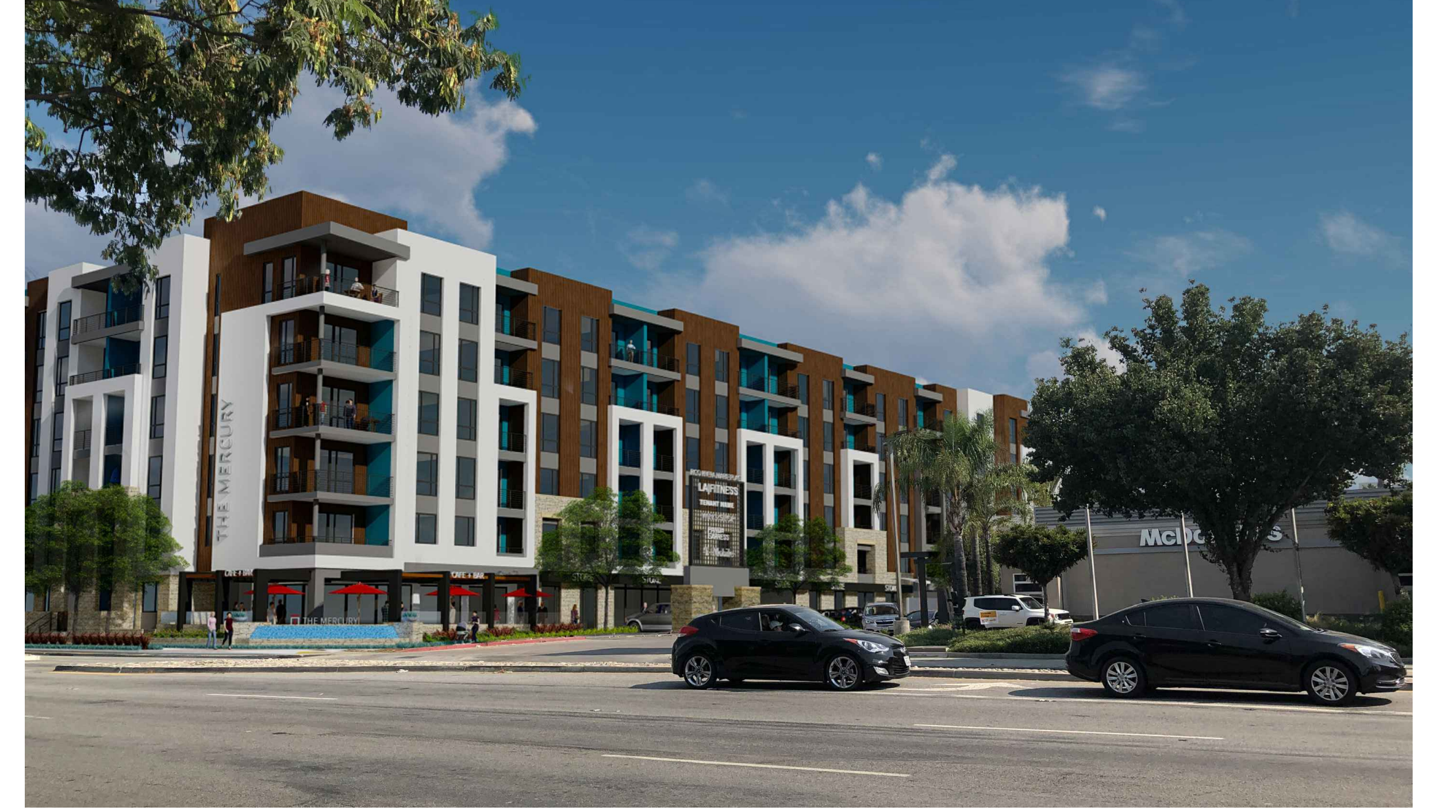
① VIEW FROM WASHINGTON AVE.
