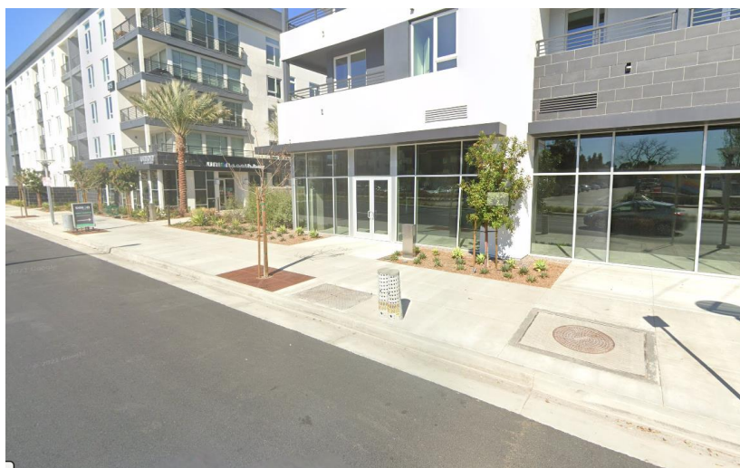
Active ground-floor frontage design on a major arterial on a recently completed project in Carson, CA. Source: Google
