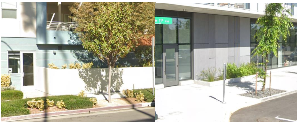
Example of raised stormwater planter (left) and recessed stormwater planter (right). Source: Google
