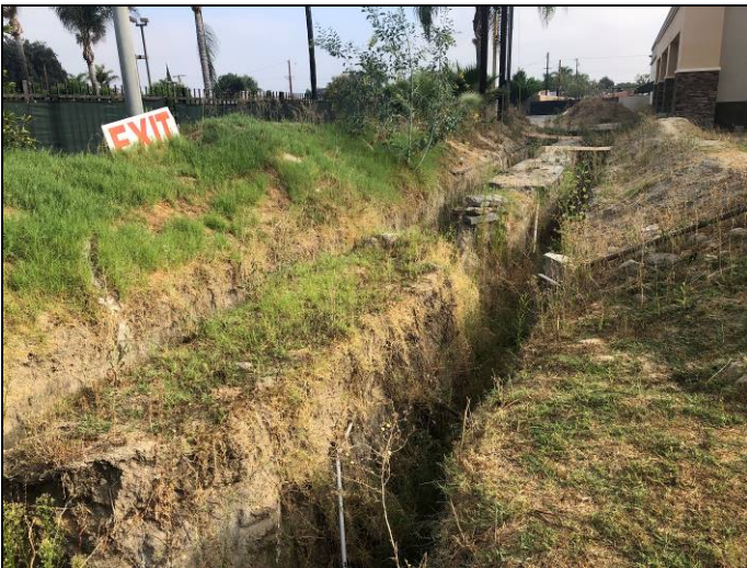
9. View of trench of subject Property
