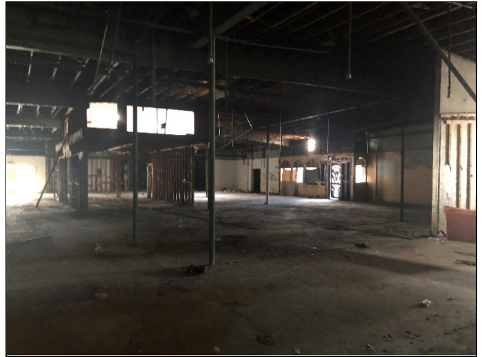
8. Interior view of subject Property structure
