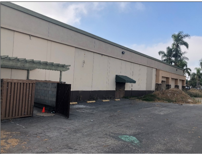
3. View of subject Property structure
