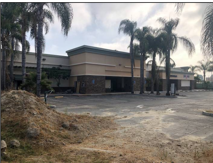
5. View of subject Property structure
