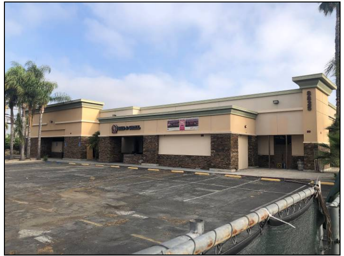
2. View of subject Property structure
