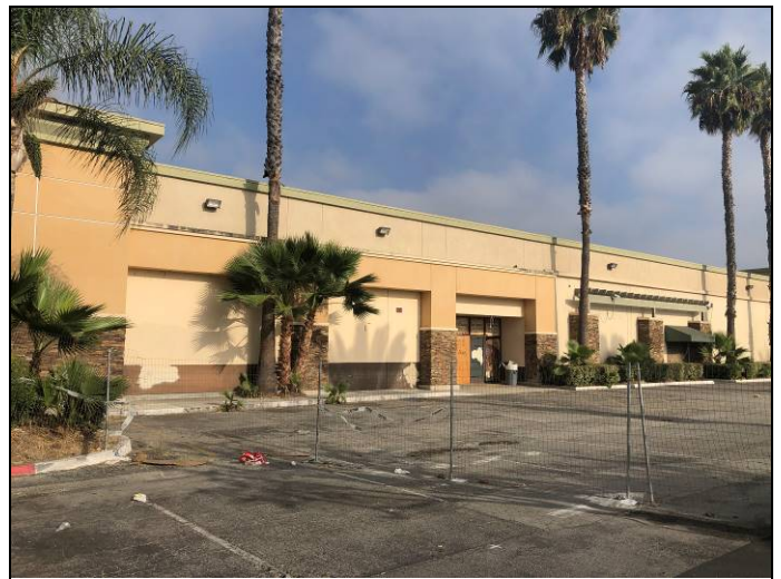
4. View of subject Property structure
