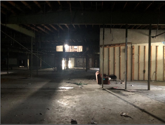
7. Interior view of subject Property structure
