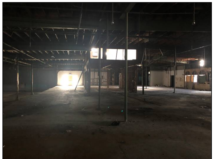
6. Interior view of subject Property structure
