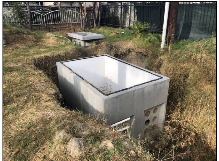
10. View of what appears to be a new greasetrap
