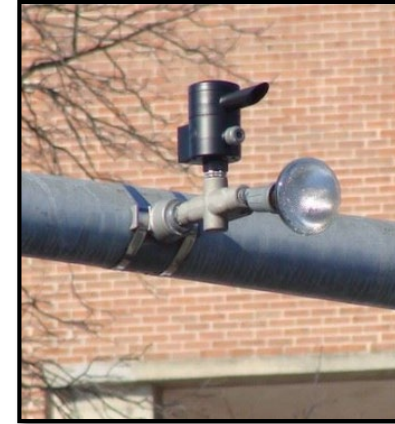
S05- Install emergency vehicle pre-emption systems
