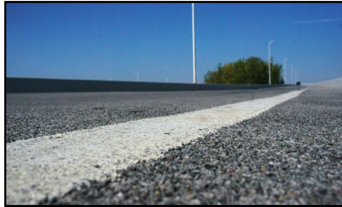
R21- Improve pavement friction (High Friction Surface Treatments)
