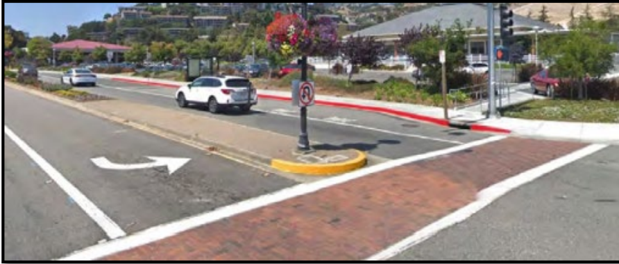
S12- Install raised median on approaches
