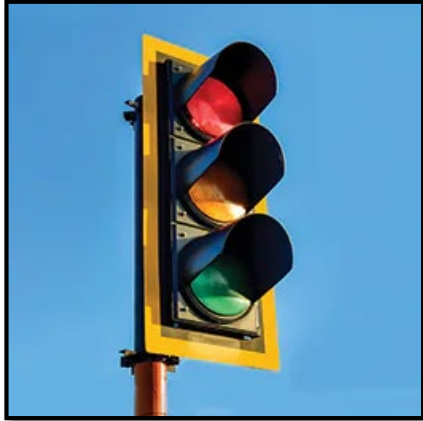
S02- Improve Signal Hardware (lenses, back-plates with retroreflective borders, mounting, size, and number )
