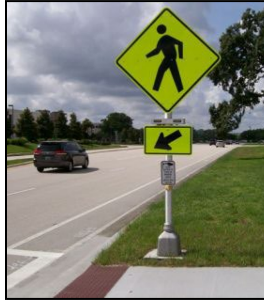
NS22PB- Install Rectangular Rapid Flashing Beacon (RRFB)
