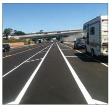
Class 2 Buffered Bike Lane - Both Sides Buffered
