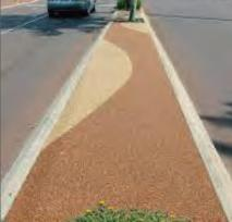
Permeable Concrete with Sand Filtration and Subsurface Drain
