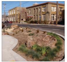
Intersection Bulbout with Bioretention Soil and Subsurface Drain
