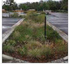
Infiltration Basin with Bioretention Soils and Subsurface Drain
