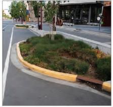
Mid-block Bulbout with Bioretention Soil and Subsurface Drain
