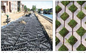
Subsurface Silva Cell and Drain (Use with Permeable Surfaces)
