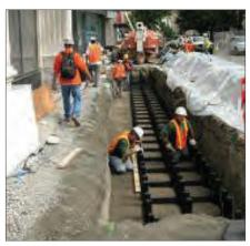
Subsurface Silva Cell with Subsurface Drain
