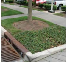
Tree Basin with Filters and Subsurface Drain
