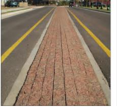
Permeable Paver with Subsurface Filtration and Drains
