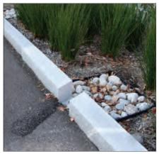
Curb Openings Draining to Bioretention, Filtration, or Infiltration Areas
