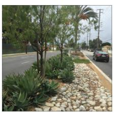
Decomposed Granite/Rock Swale/ Gravel Trench
