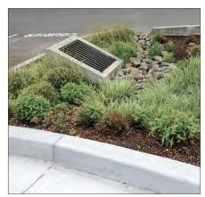
Bulbout as an Infiltration Basin with Bioretention Soils and Subsurface Drain
