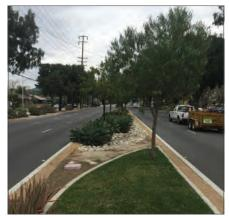
Tree Basin with Bioretention Soils and Subsurface Drain
