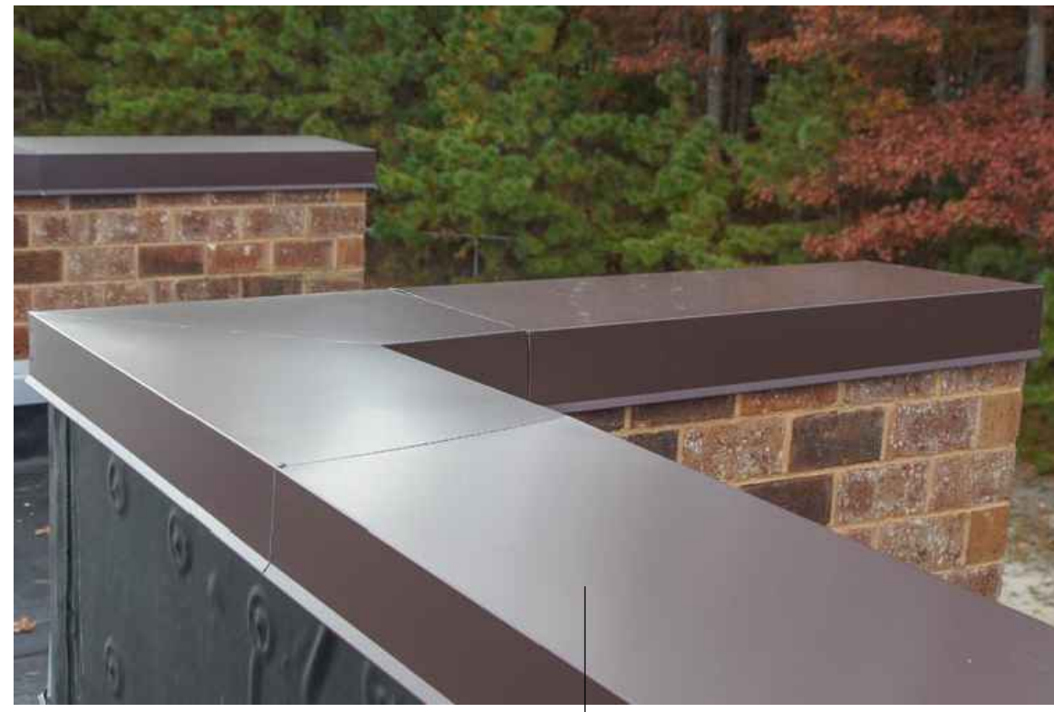
METAL COPING MFT: PAC-CLAD PRODUCT: STEEL COMPOSITE PANEL DARK BRONZE POWDER COAT
