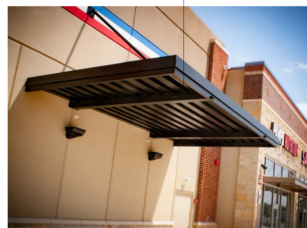
METAL PANEL CANOPY MFT: PAC-CLAD PRODUCT: STEEL COMPOSITE PANEL DARK BRONZE POWDER COAT
