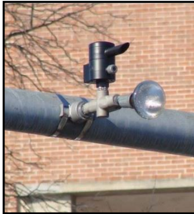
S05- Install emergency vehicle pre-emption systems
