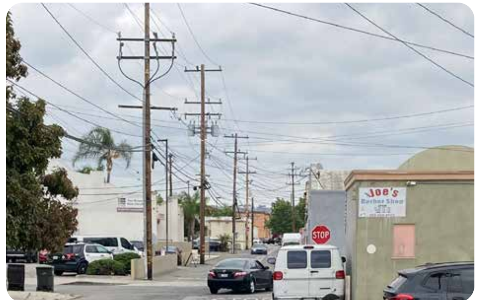
Overhead electric lines along Speedway Alley are a candidate for undergrounding as part of current planning to turn the alleys into paseos.
