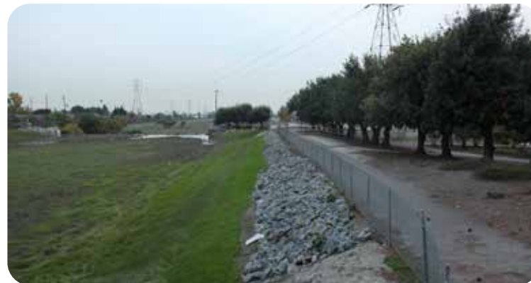
Recycled Water Turnouts (Potential Regional Park)
