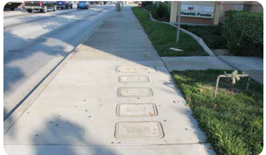
Access to water lines serving shopping centers on the south side of Whittier Boulevard along the sidewalk and parkway areas.
