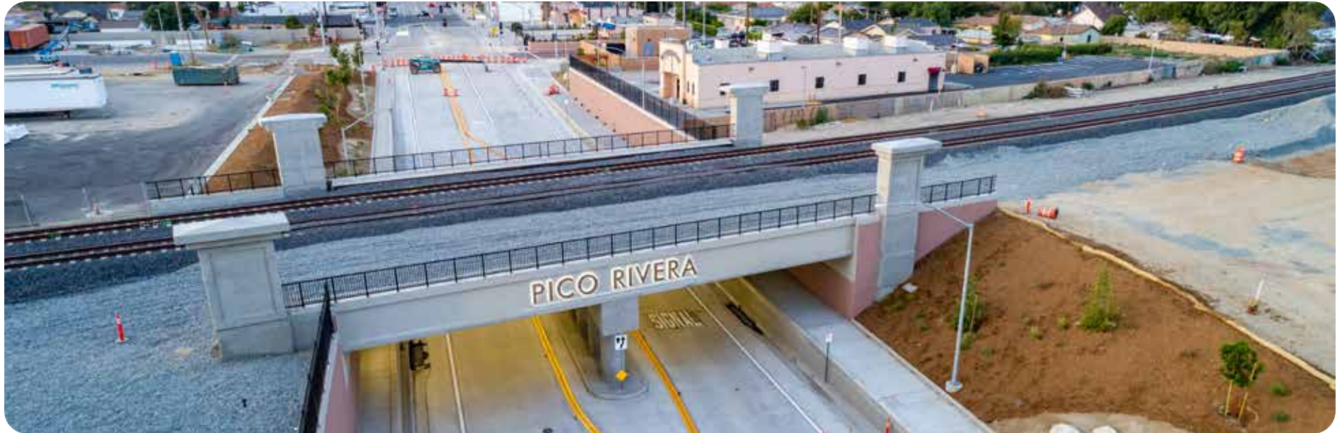
Updated rail bridge over Durfee Ave with option for adding third track.
