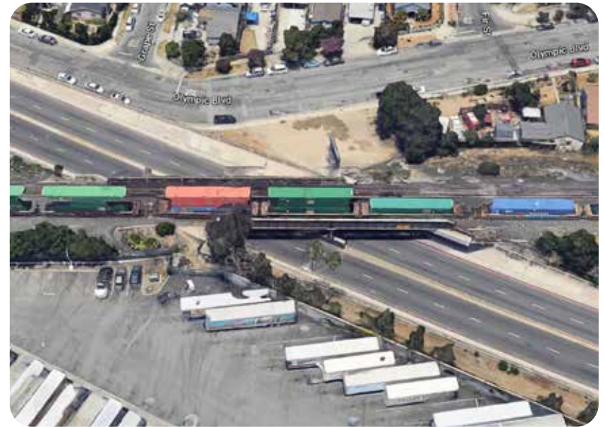
Existing rail bridge over Whittier Blvd with no room for third track and bridge supports encroaching upon sidewalk area under bridge.
