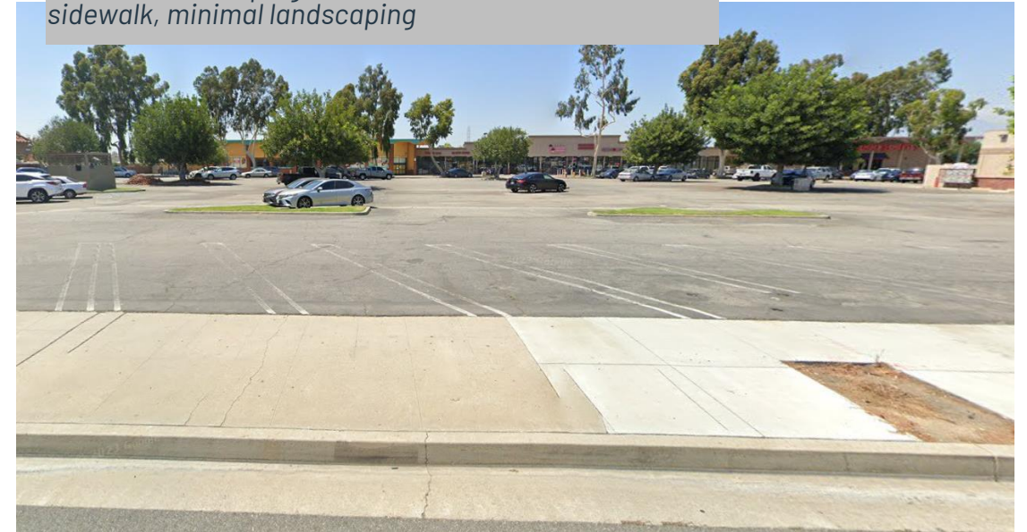
Wheel stops, pedestrian pathway, stormwater capture, lighting, defined striping
