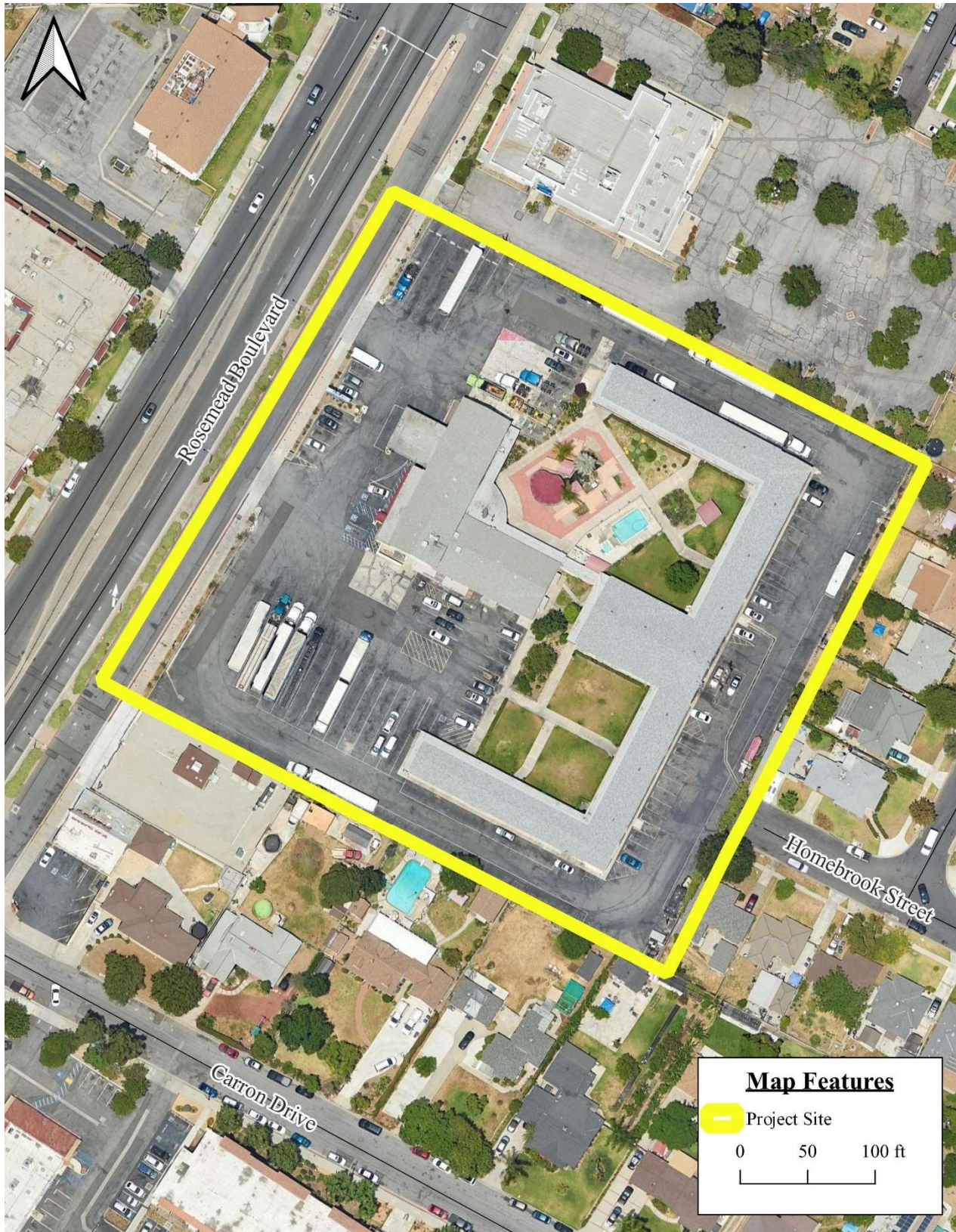
EXHIBIT 4 AERIAL PHOTOGRAPH Source: Google Maps
