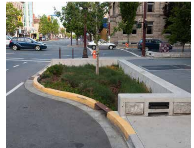
Example of permanent curb extension with a bioswale, street tree, and pedestrian seating, which could be upgraded from a painted curb extension completed in Phase I
