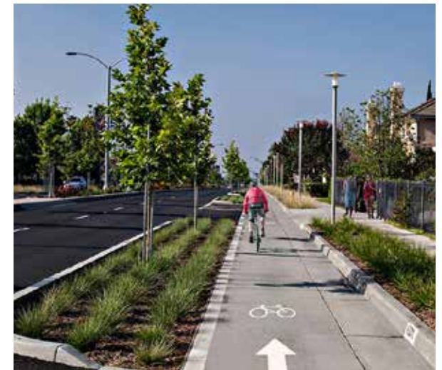
Example of bioswale protected bicycle lane along Rosemead Boulevard in Temple City, which provides a case study for the development of the same facility along Whittier Boulevard due to similar roadway designs, traffic volumes, and adjacent land uses.
