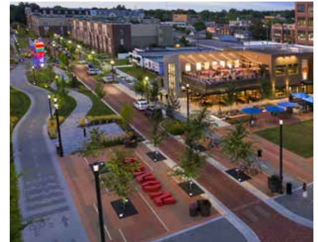
A block of the Indianapolis Cultural Trail demonstrates how different pavement materials indicate different uses for the street right-of-way and integrates with adjacent buildings to create attractive outdoor dining spaces.
