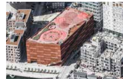
P3 parking structures for public parking and catalyze new development
